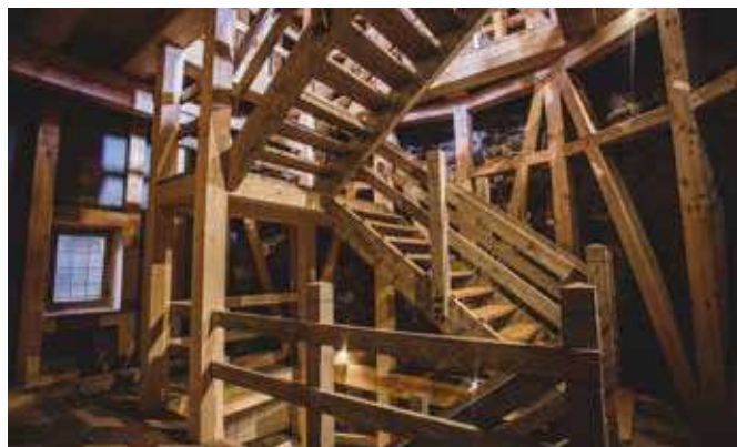
Torņa trīs stāvi savienoti ar atklātām iekšējām koka kāpnēm. The three floors of the tower are connected by an open internal wooden staircase.
