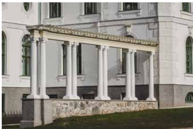
No jauna izgatavotas pergolas kolonnas. The columns of the pergola are newly made.
