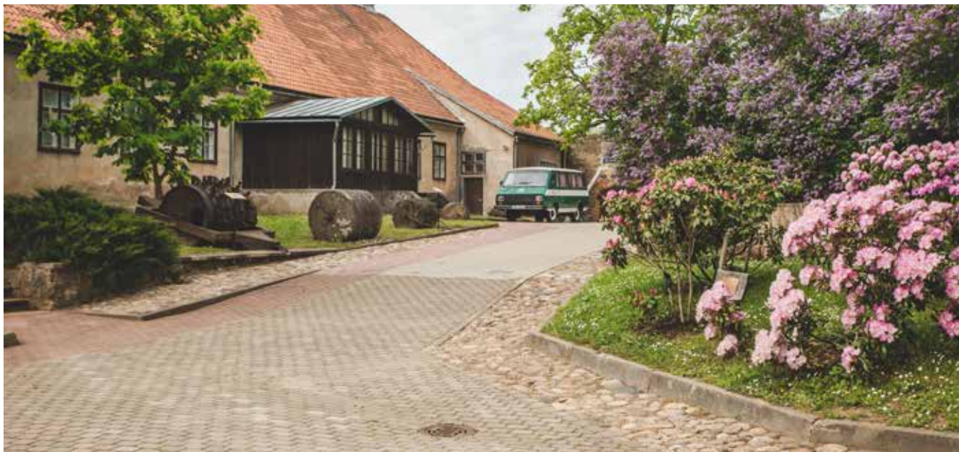
Muižas pagalmā ieklāts bruģis. Muižas ēkai atjaunots dakstiņu jumta segums. Paving is laid in the courtyard of the manor. The tiled roof of the manor house is restored.
