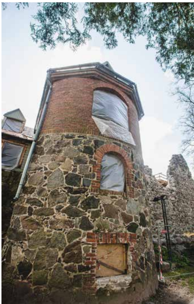
Konservē un restaurē Valmieras viduslaiku pils daļu. A part of the castle is being restored and conserved.
