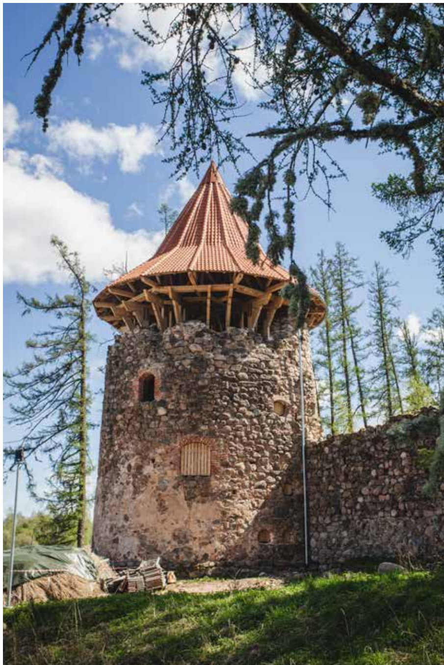
Restaurēts un atjaunots pils Ziemeļu tornis. The Northern tower of the castle is restored and renovated.
