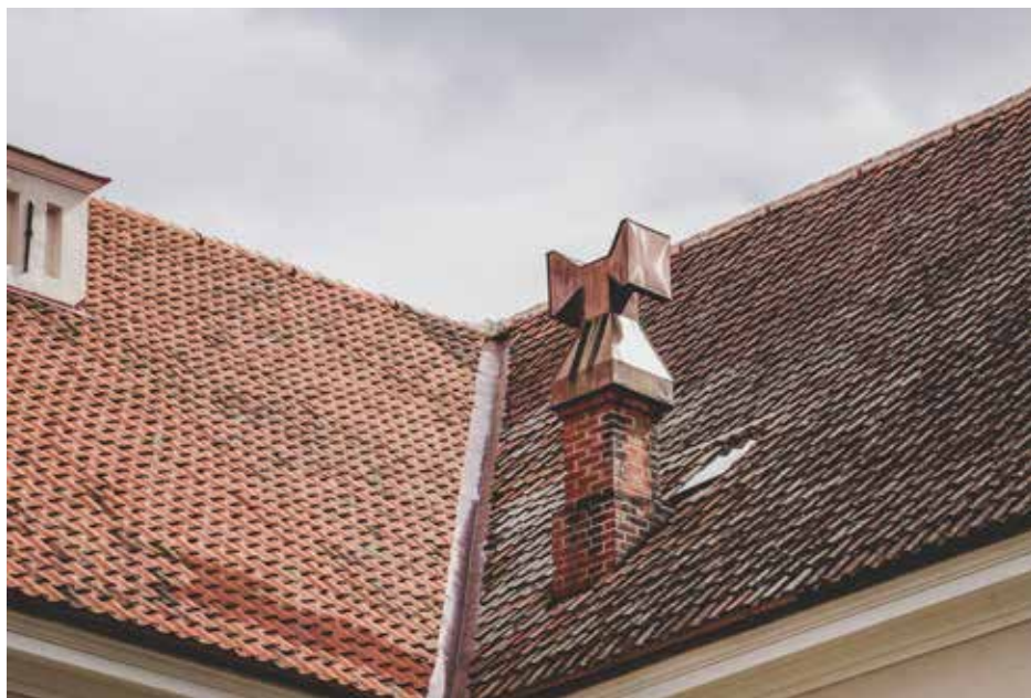
Atjaunots baznīcas jumta segums. The church roof is renewed.
