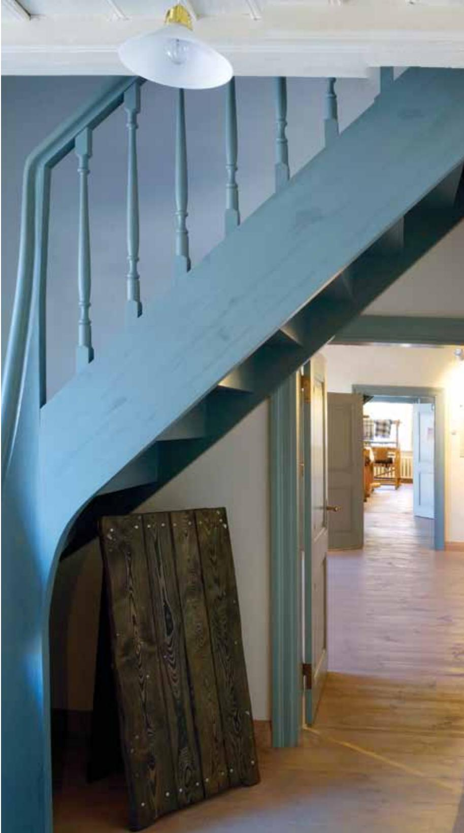
Traditional methods and natural materials were used in the restoration. Construction elements such as floors, stairs, window shutters and doors were manufactured at the local Rumba carpenter's shop. Lime mortar and lime paint were used for to decorate the interior walls, wooden parts were painted using linseed oil paints produced at a local workshop, the façade was caulked using tar-soaked tow and painted using natural tar paint.
